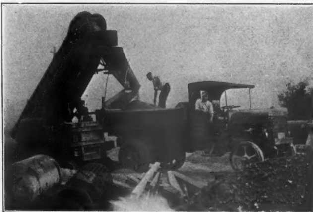
Loader Reclaiming Crushed Rock from Ground Storage
